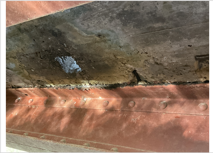
Exposed reinforcing steel in the deck soffit adjacent to the deck drain. Beam # 1.
