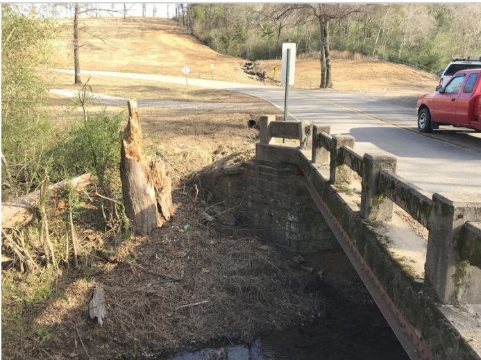
Stone displacement in wing wall at Bent 2 left.
