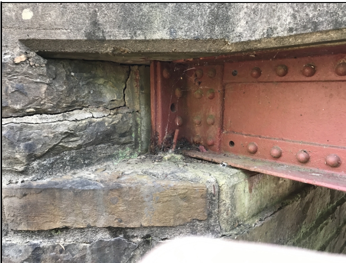
Bent # 2, Beam # 1 active corrosion.
