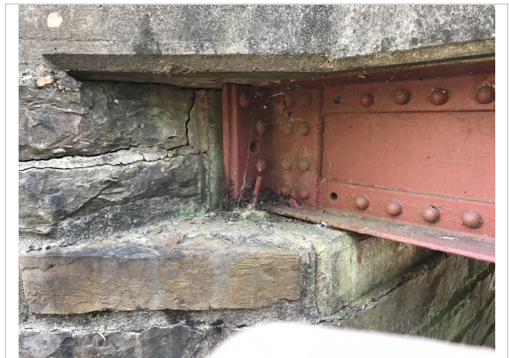
Bent 2 ,beam 1 active corrosion.
