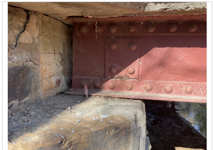
Bent # 1. Beam # 10 corrosion.
