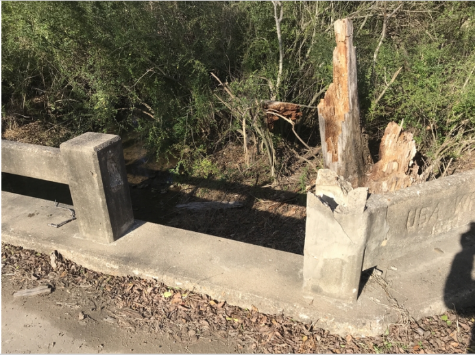
Northeast corner bridge rail damage.
