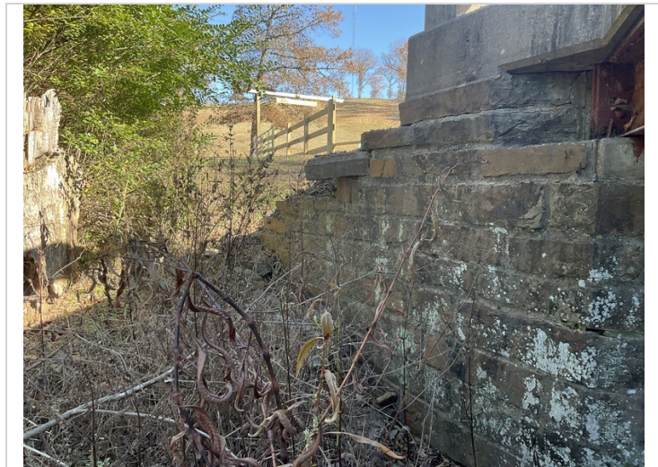
Northeast wing wall. Stone displacement.
