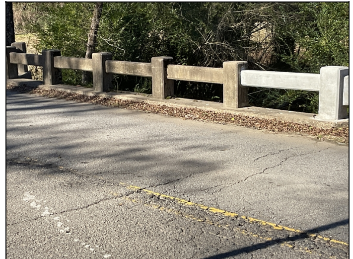
Debris accumulation in the gutters.
