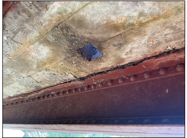
Beam # 10 corrosion adjacent to the deck drain.
