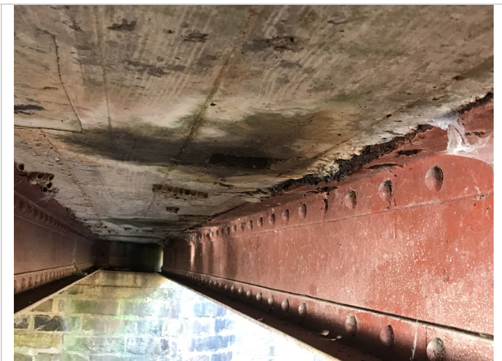
Beam1 active corrosion near the deck drains.
