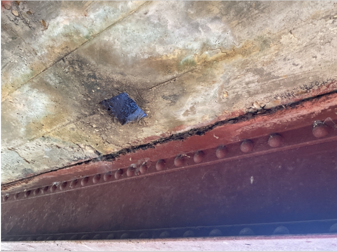
Beam # 10. Corrosion adjacent to the deck drains.
