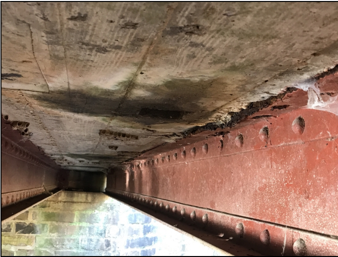
Beam # 1 active corrosion near the deck drains.
