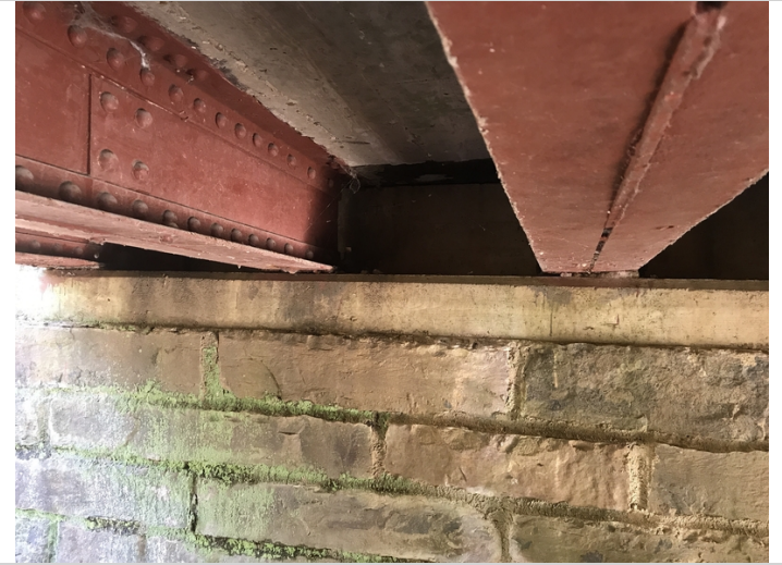
Bent 2 ,beams 2 and 3 pack rust between the cap and the bottom flange of the beam.
