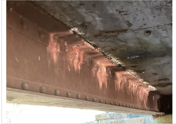
Beam # 1 - beam corrosion adjacent to the deck drain.
